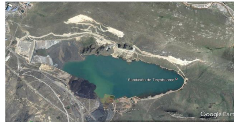
El Brocal's Modern Downstream Tailing Dam
