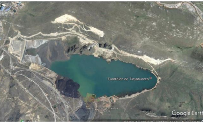
El Brocal's Modern Downstream Tailing Dam
