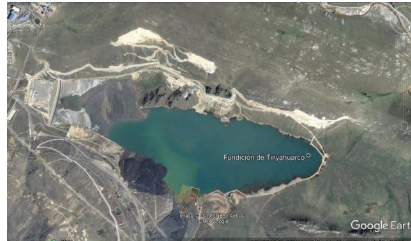
El Brocal's Modern Downstream Tailing Dam
