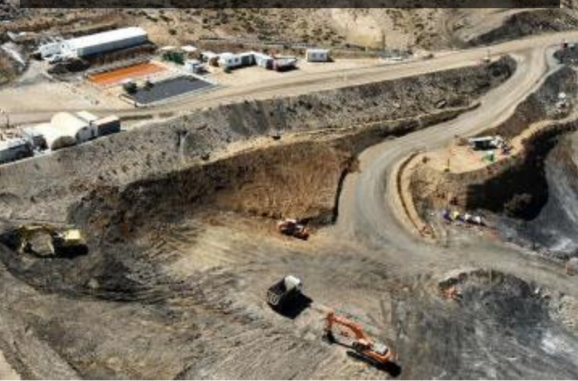
Mine Pond & Industrial Treatment Water Plant earthworks.
