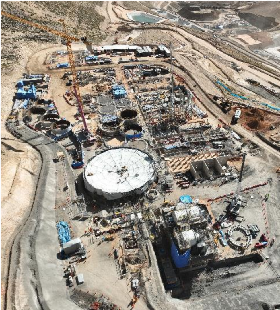
Processing Plant: 80% Progress on Foundations
