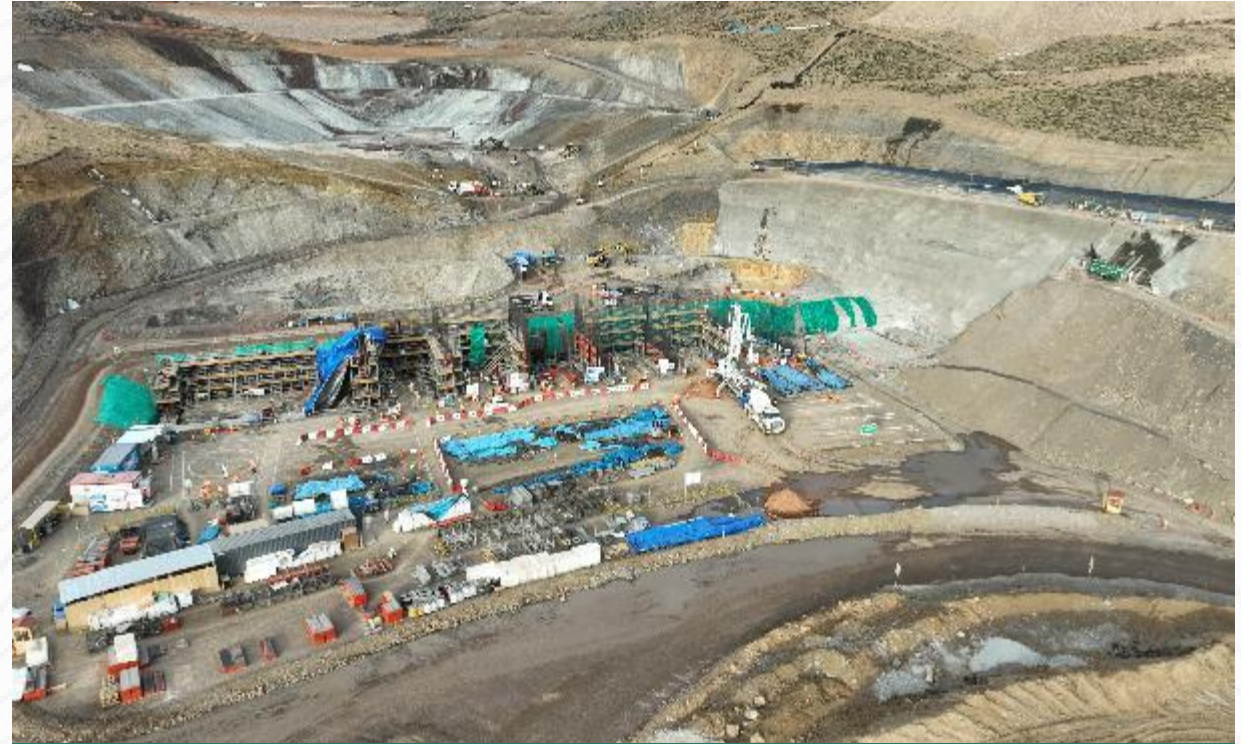
Filtering plant civil works
