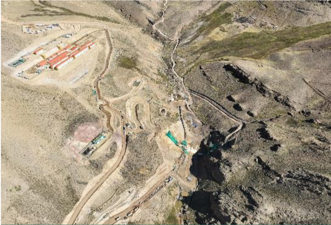
Water dam foundation completed
