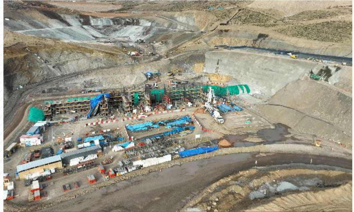
Filtering plant civil works
