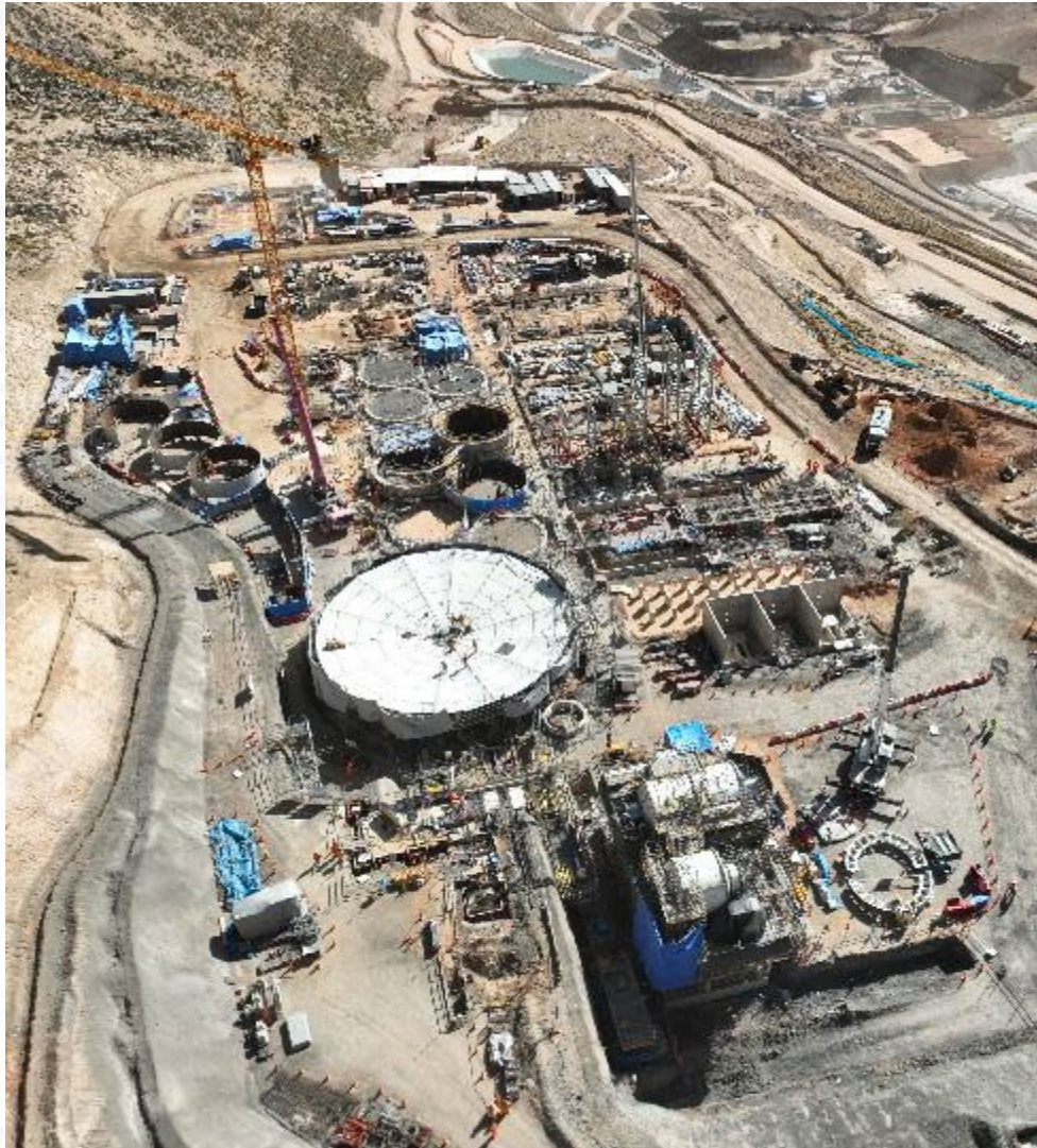
Processing Plant: 80% Progress on Foundations
