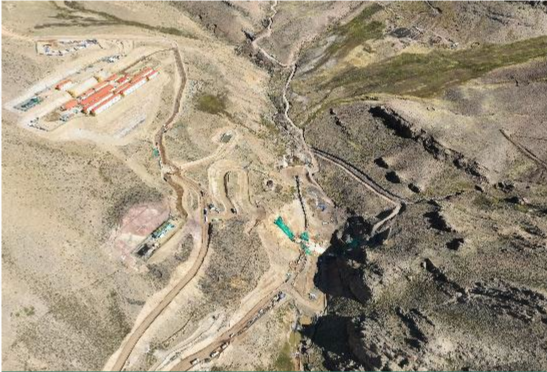
Water dam foundation completed
