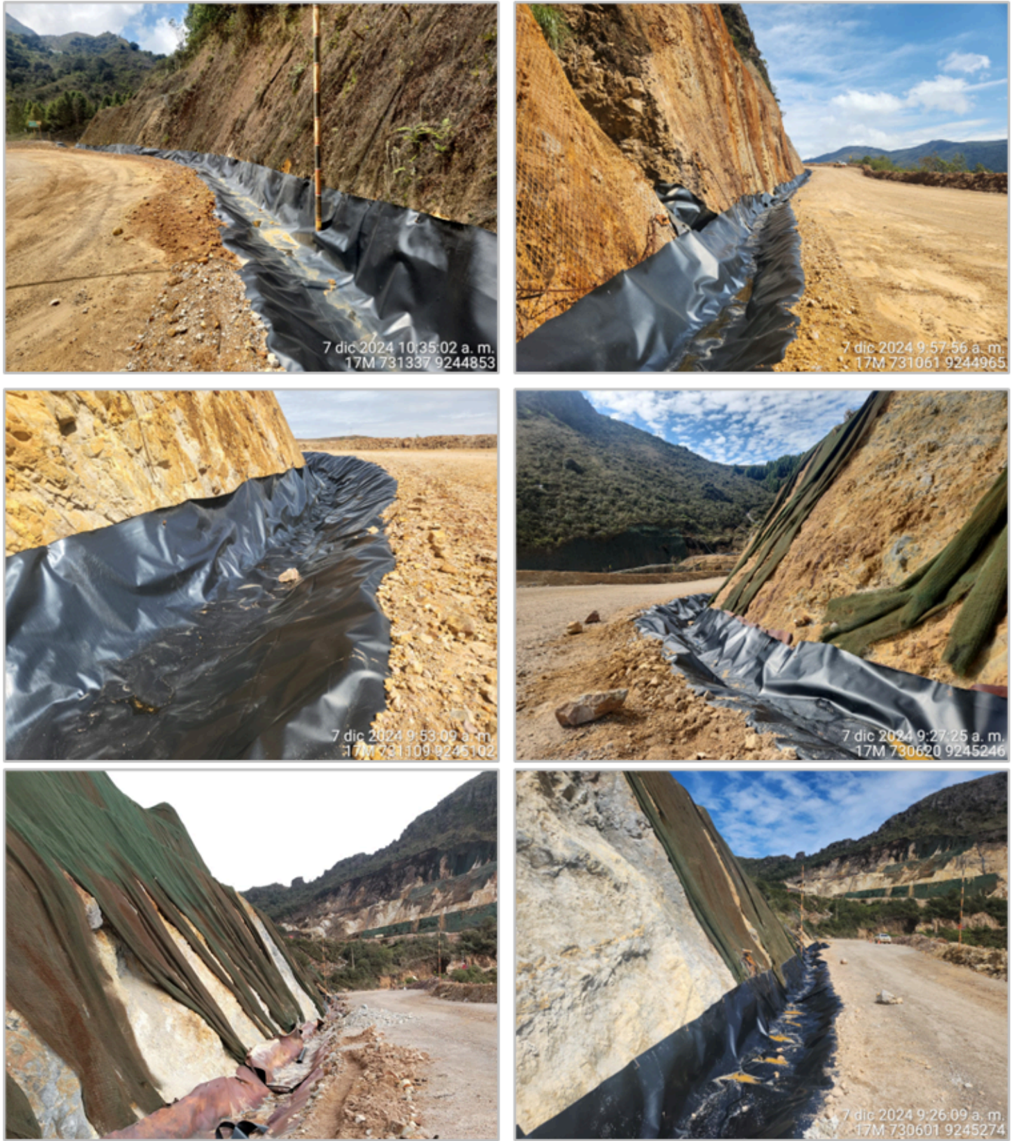
Cleaning and lining of canals
