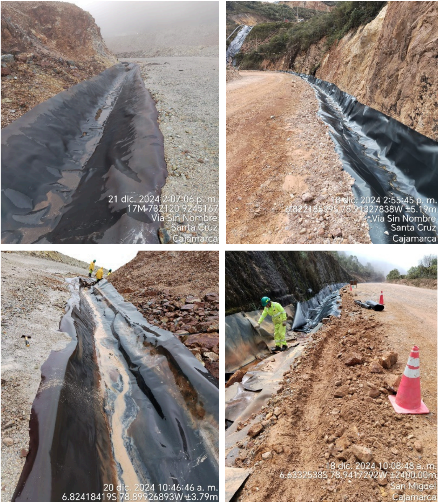
Cleaning and lining of canals
